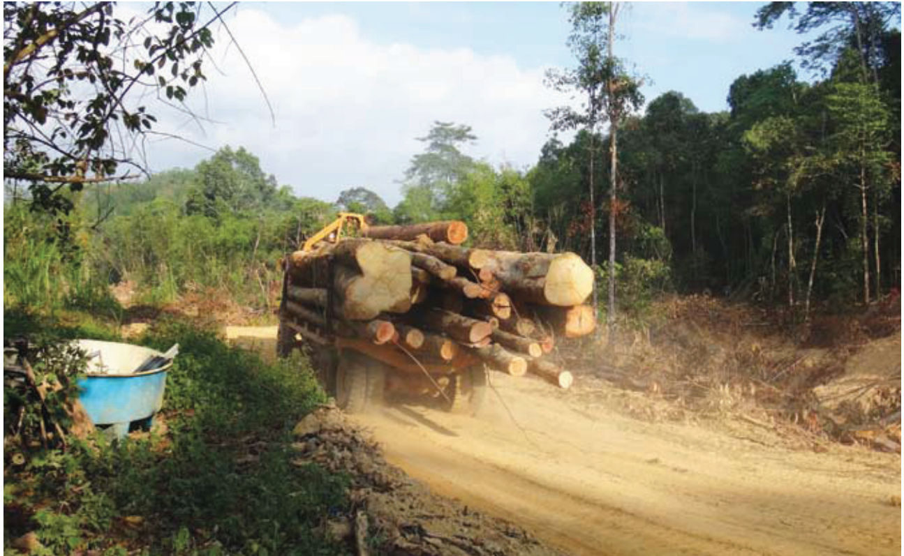
Log extraction at the back of the farm that has caused soil erosion and water pollution and posed a serious threat to the farm
